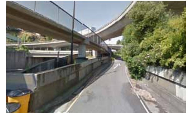
Existing Conditions: Motorists' perspective from Highway 101 off-ramp. Drivers can not see the crosswalk (shown in photo on left) less than 160 feet ahead.
