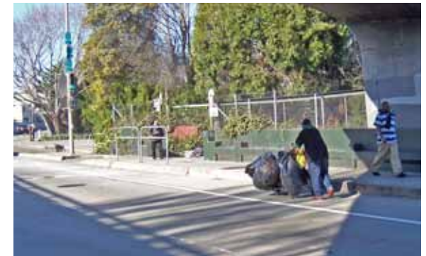
Existing conditions at the northern portion of segment D. Note pedestrian in bicycle lane and tight spacing of sidewalk, railings, fences and curb ramps.
