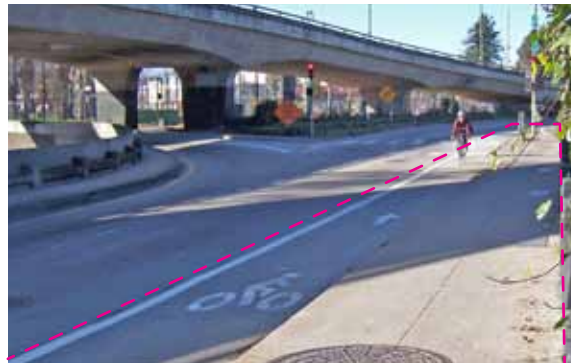
Existing conditions with location of recommended two-way multi-use path outlined. Note southbound cyclist in northbound bicycle lane.
