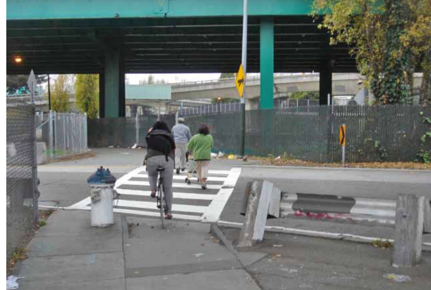
Existing conditions, east end of segment J looking west to segment I. Traffic approaches from the left. Note lack of maneuvering room and visibility.
