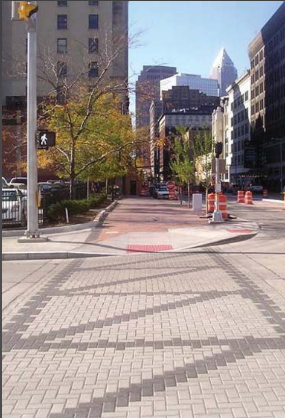
Pavers in crosswalk
